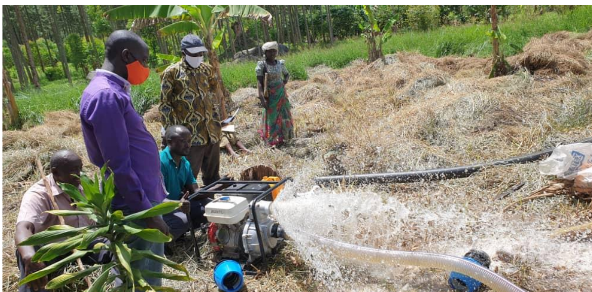
Installation of the irrigation pump at LSB Kitembe
